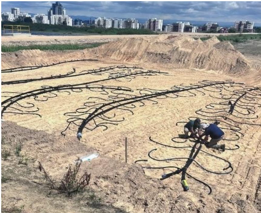
Figure: Installation of a piping system
